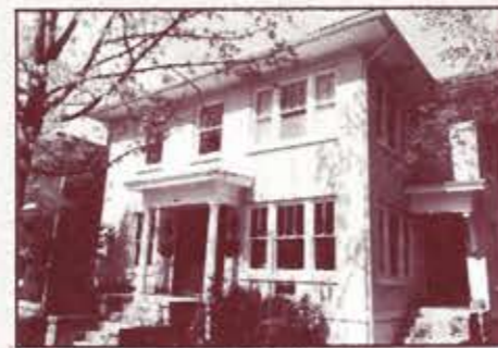
1 ARTHUR G. RUSSELL HOUSES 544-548 EAST MAIN STREET Two of Bowling Green's early duplex houses were built circa 1924 by Arthur Russell, a local lumber dealer.
